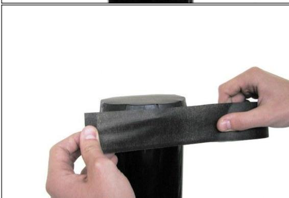
**Tape the edge of the pressure cap with the special pressure cap tape.**
